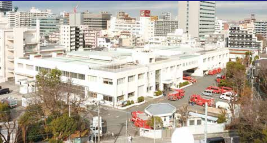
◀ Present view of the Maintenance Shop
